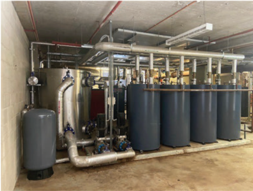
Hot & Warm Water System Maintenance Repair and Replacement
