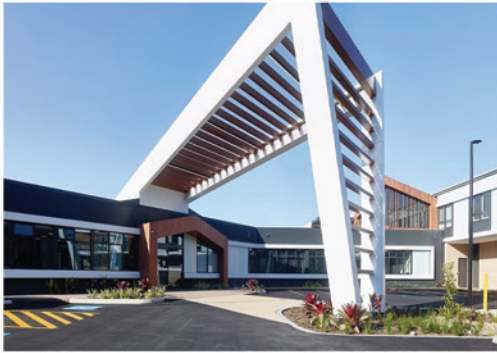
Plumbing, Draining & Gas Maintenance
